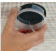
1. Cut hole and mount flush mounting clip
