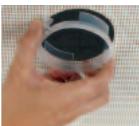
1. Cut hole and mount flush mounting clip
