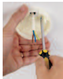
1. Mount surface box onto the ceiling, and remove minitrunking knockout
